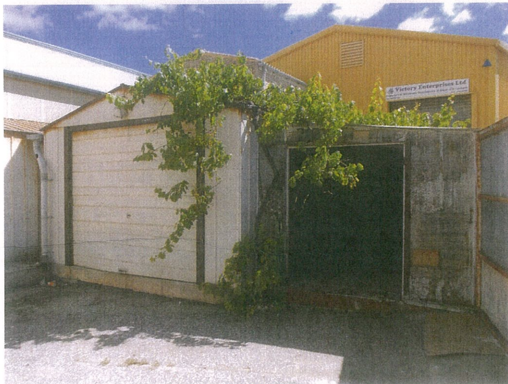
Fig 4 Building No 3 and No4
